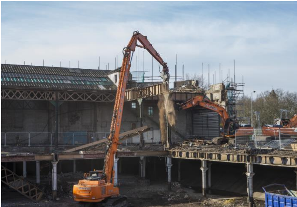
Photo of demolition works – Former Rosa Freedman Centre
